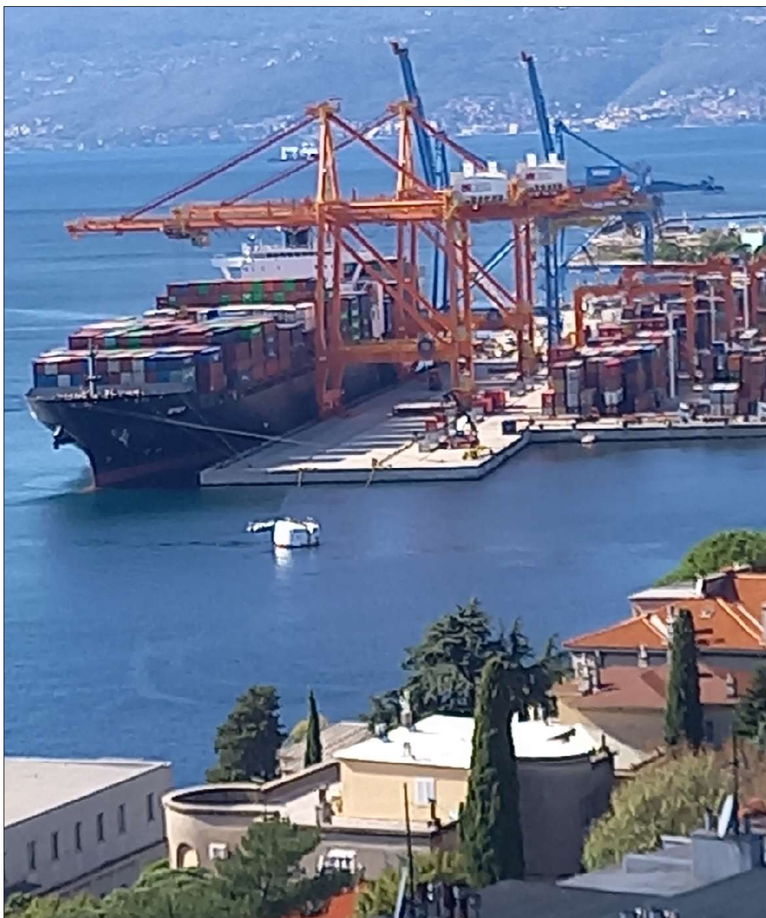
Slika 5 - AGCT Rijeka - International Containet Terminal Services
