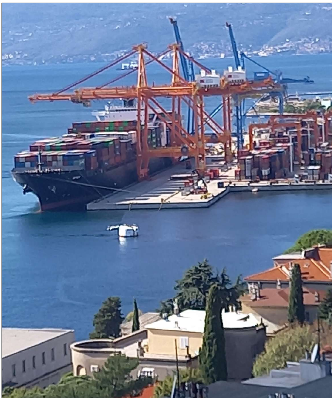
Slika 5 - AGCT Rijeka - International Containet Terminal Services
